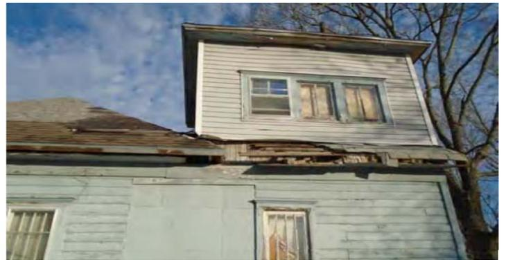
**(Top)** This home has a collapsed roof and seven layers of shingles. **(Above)** Broken windows and a damaged roof were among the problems associated with this structure.
